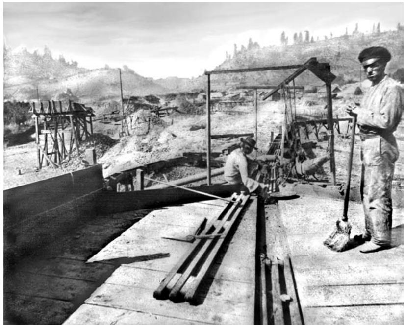
Placer Mining at Volcano. Cleaning up the dump box, mid 1860s.
